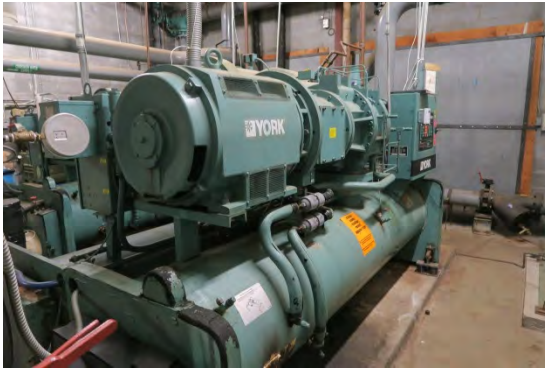
Chillers (1 and 2) in mechanical penthouse
