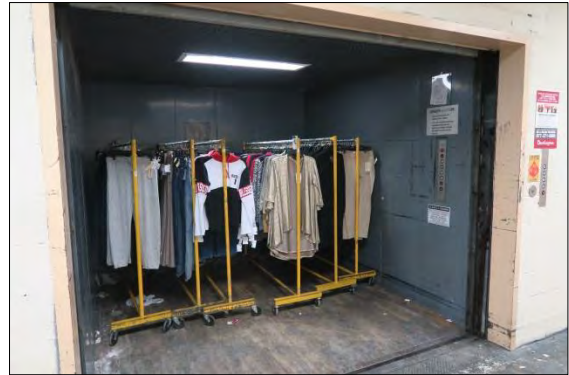
Interior of freight elevator
