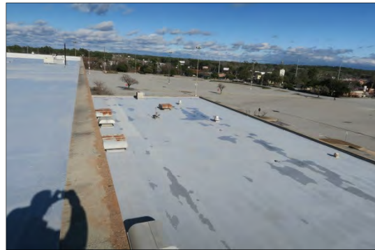
Lower roof at auto shop area
