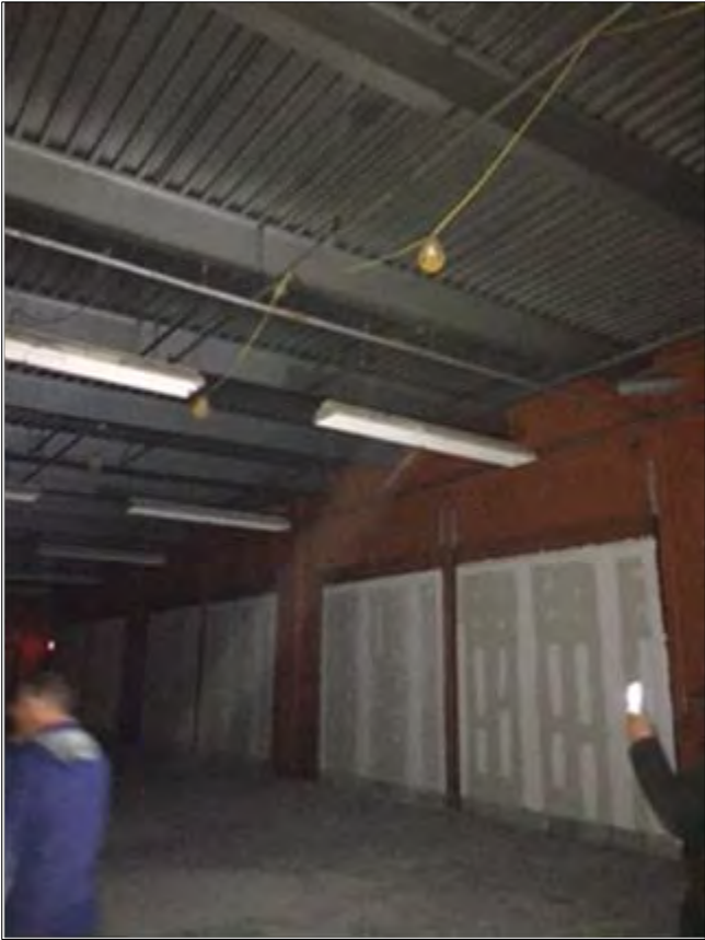
Structural construction in old auto bays
