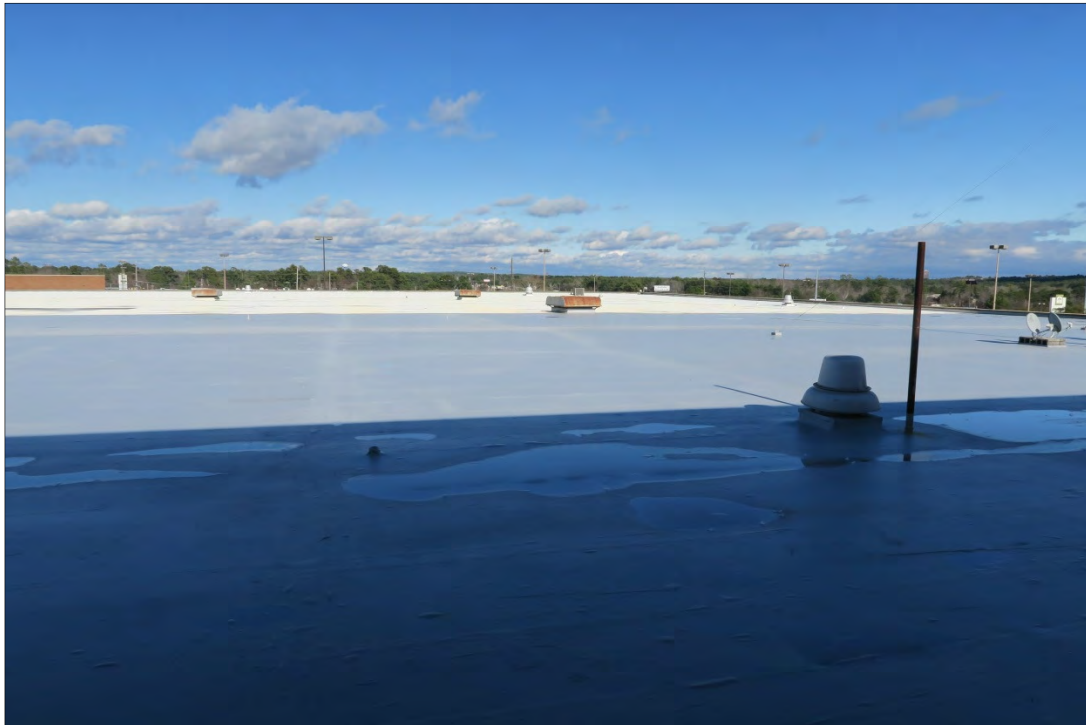
Roof showing the two different areas (the treated-gray and untreated areas-white)
