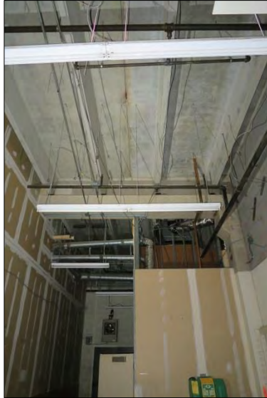
Double "T" structure in storage area
