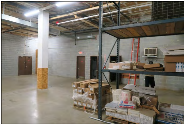
Structural column and drywall covered decking @ storage area
