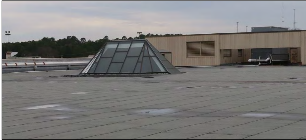
Skylight at atrium
