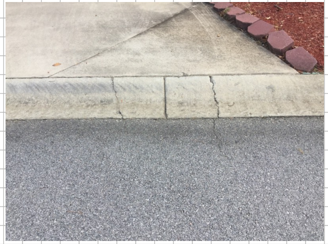
Heavy damage on curb approximately 1.5'
