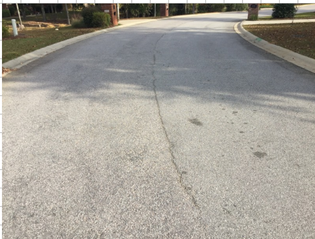
Cracking forming at crown of road and approximately 141' starting at address 427 to 435. Along the crack in crown of road, potholes and alligator cracking has started to form near address 435, approximately 9' x 1'
