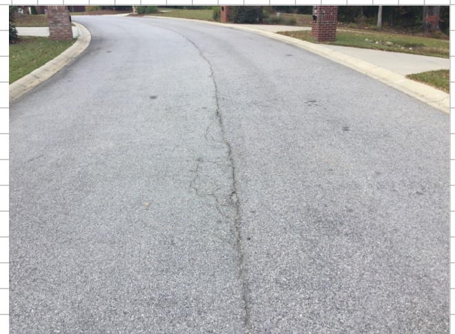
Cracking forming at crown of road and approximately 141' starting at address 427 to 435. Along the crack in crown of road, potholes and alligator cracking has started to form near address 435, approximately 9' x 1'
