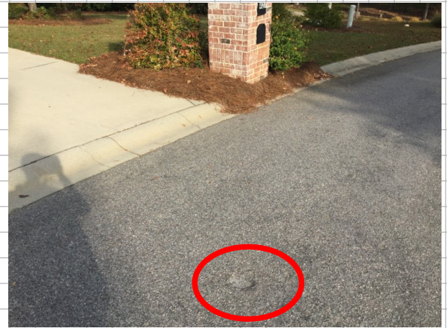
Small pot hole forming at address for 427 and outbound lane
