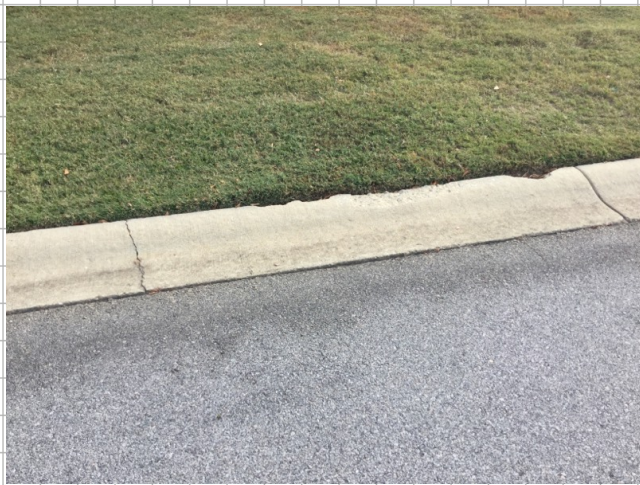
Example of curb damage found throughout subdivision.
