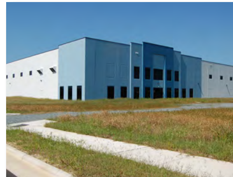
Monroe-Union County Spec Building 109,000 SF, Monroe, NC
