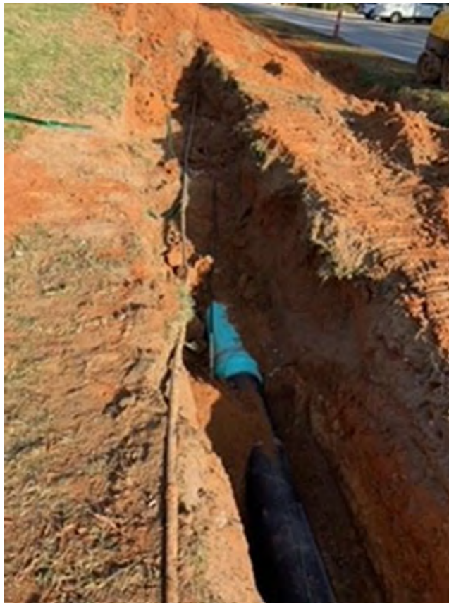
Photo 4: Force main install
