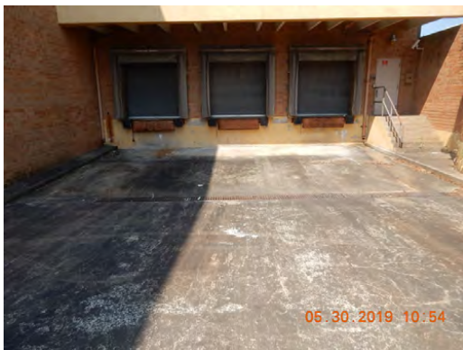
Dock, exterior steps, lighting
