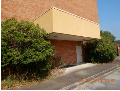
Service door, cladding
