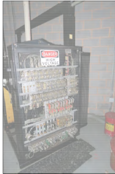
Controls for glass elevator
