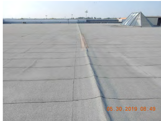
Roof expansion joint
