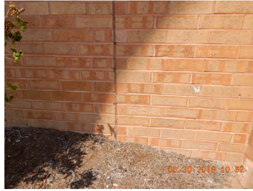
Control joint sealant
