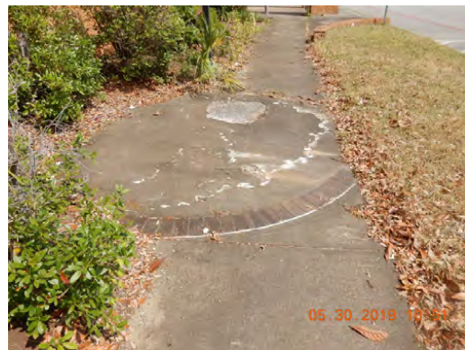
Sidewalk spall
