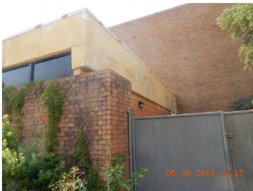
Cladding at dock
