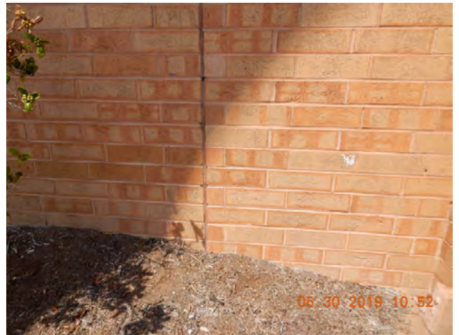
52. Control joint sealant
