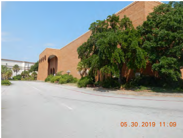
11. Drive aisle, south elevation landscape
