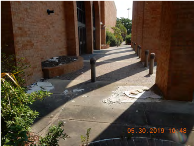
61. South entry sidewalk
