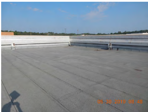
Roof, parapet, area drainage
