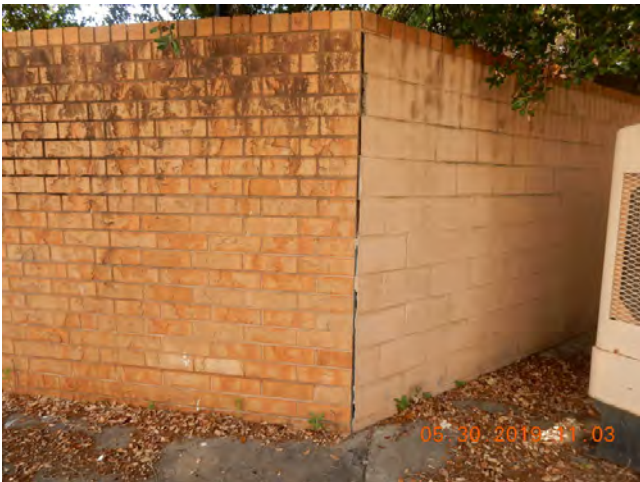
23. Perimeter wall, north elevation
