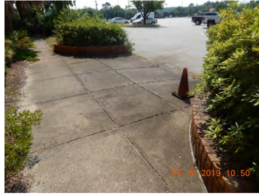
Sidewalk, curb ramp
