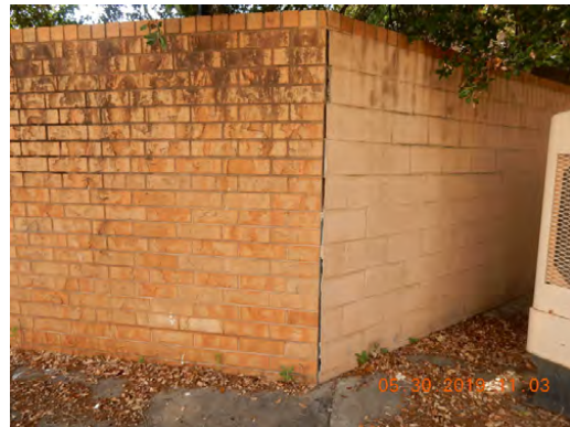
Perimeter wall, north elevation
