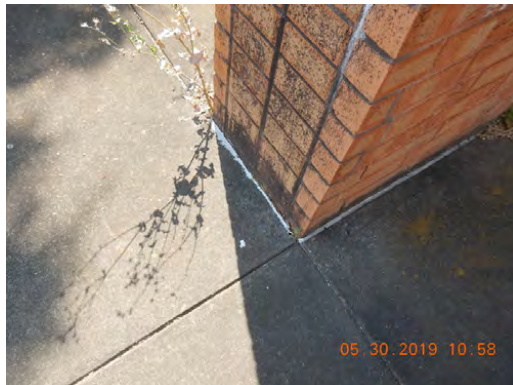
Sealant at foundation line
