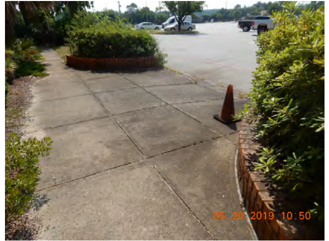
58. Sidewalk, curb ramp
