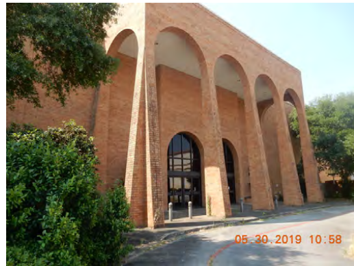
North elevation entry
