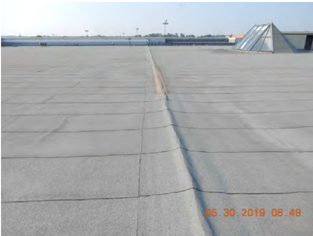
131. Roof expansion joint
