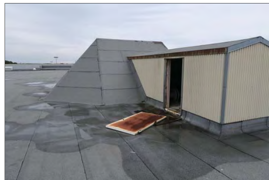
Roof at skylight with some ponding
