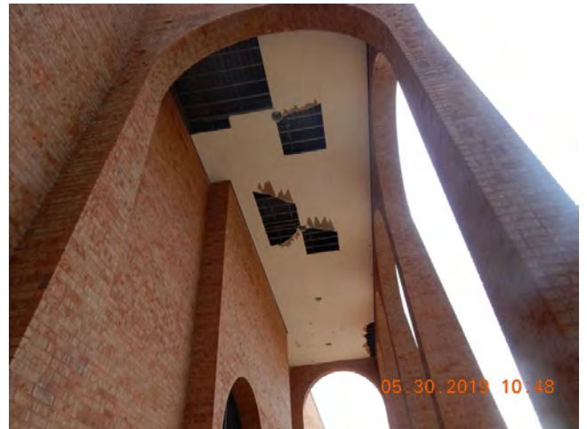
60. Soffit, south entry
