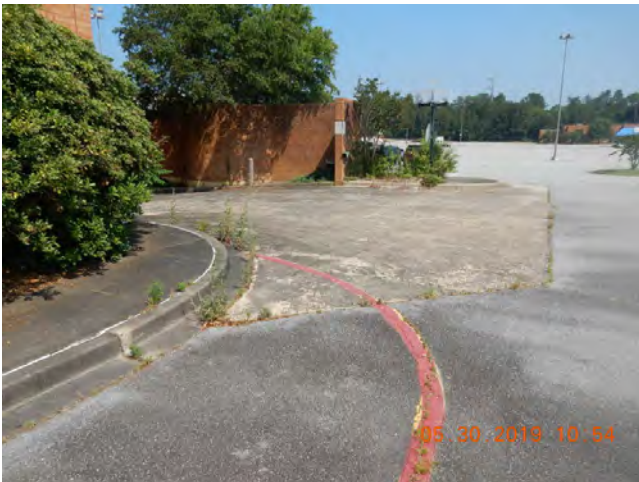
47. Curb, gutter, dock apron
