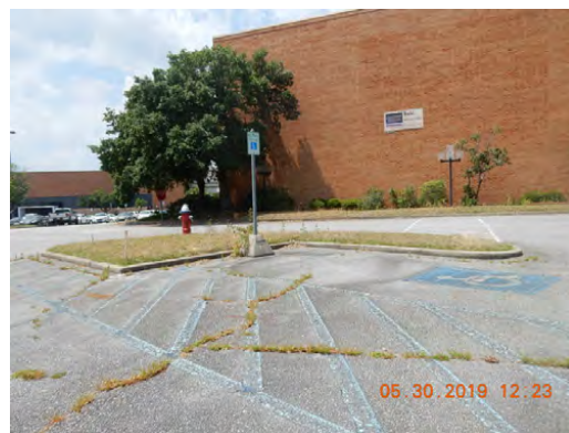
Paving, designated parking
