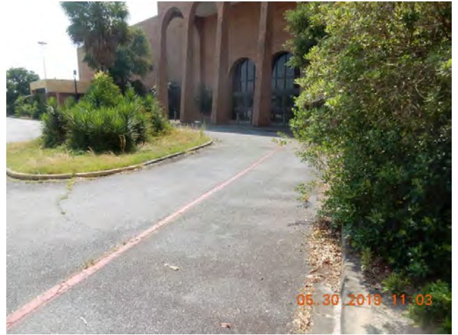
22. Drive aisle, landscape island
