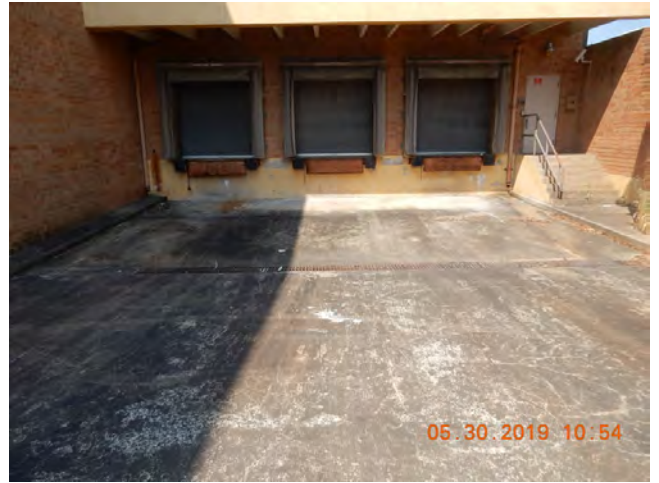
46. Dock, exterior steps
