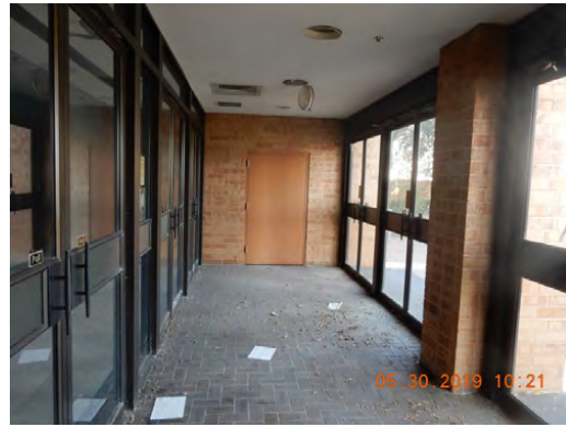
Entry vestibule, security screen left, above
