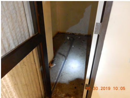
Mall common entry door track
