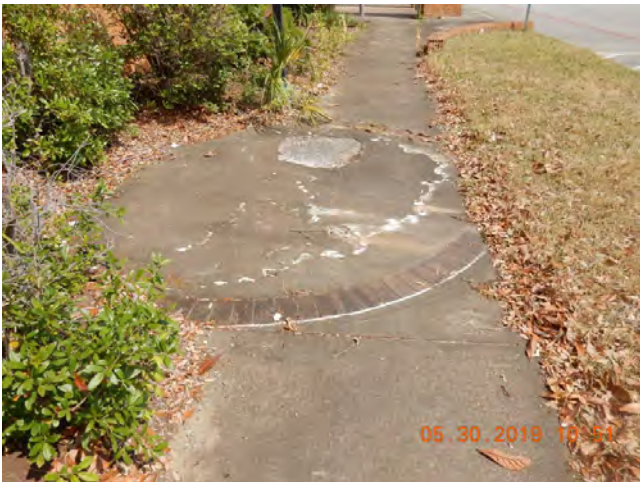
55. Sidewalk spall
