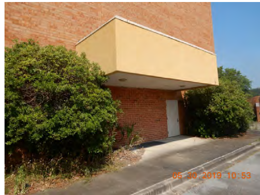
Service door, cladding
