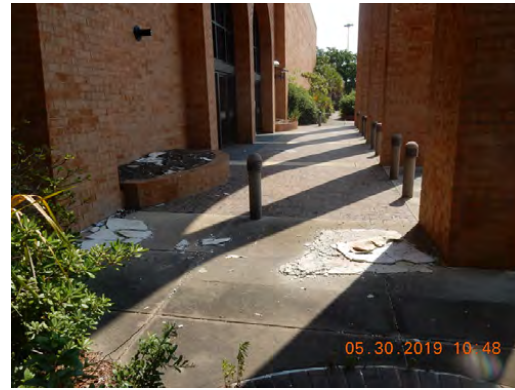
South entry sidewalk soffit sheathing
