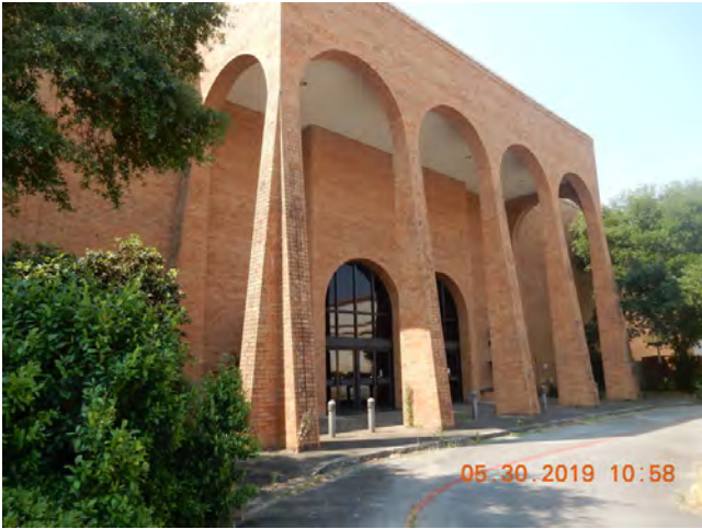
37. North elevation entry
