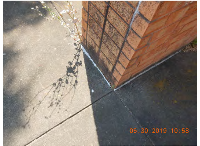
34. Sealant at foundation line
