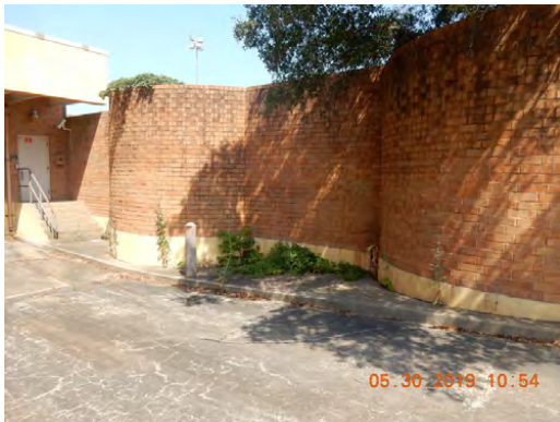
Perimeter wall at dock
