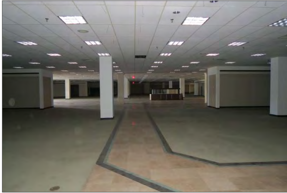
First floor space
