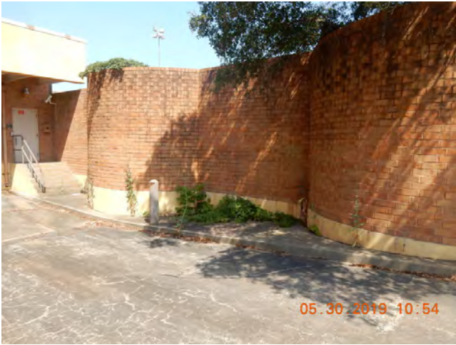
45. Perimeter wall at dock
