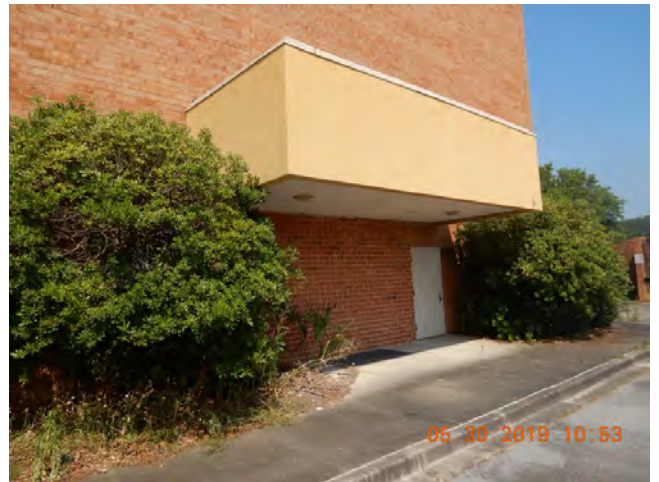
48. Service door, cladding
