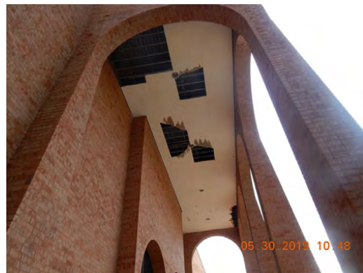
Soffit, south entry
