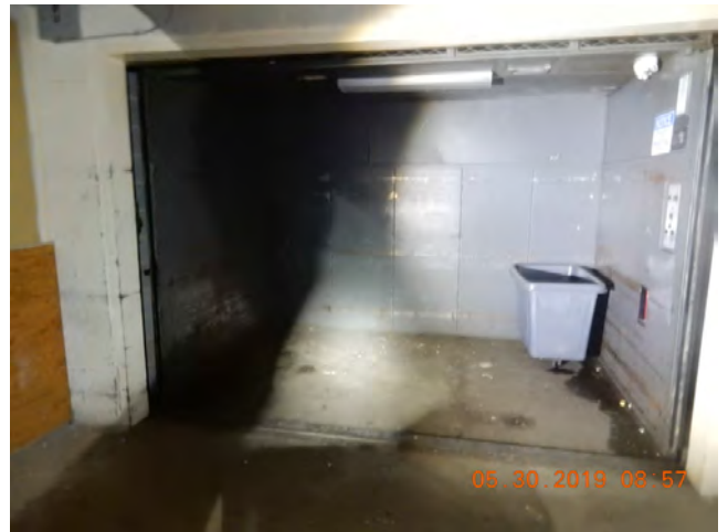
180. Freight elevator finishes
