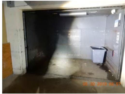
Freight elevator finishes
