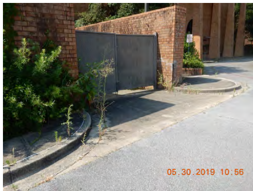
Compactor enclosure gates
