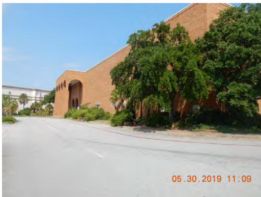
South elevation landscape
