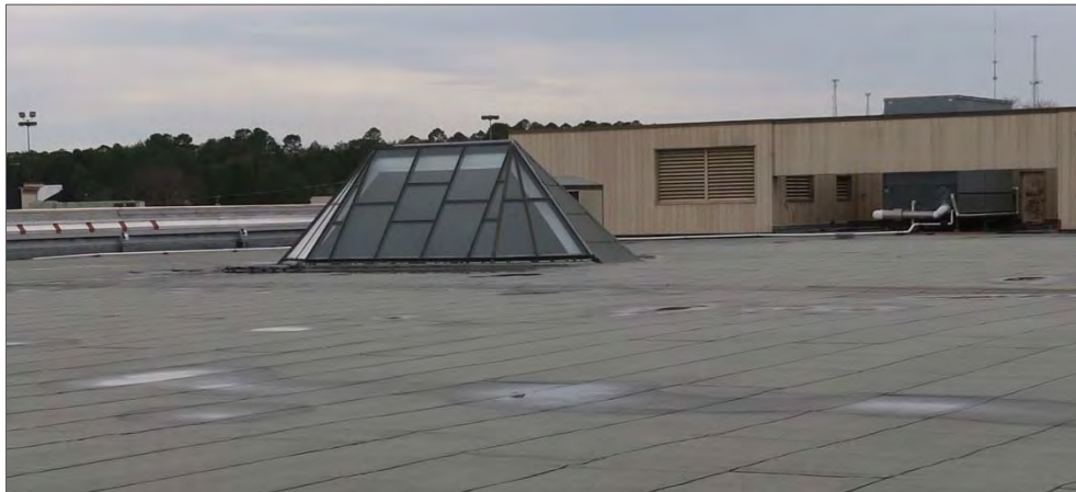
Skylight at atrium
