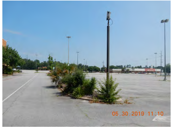
10. Site lighting, landscape island
