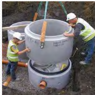
Installation of Manhole
