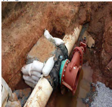
Tapping Sewer Line for Service Connection
