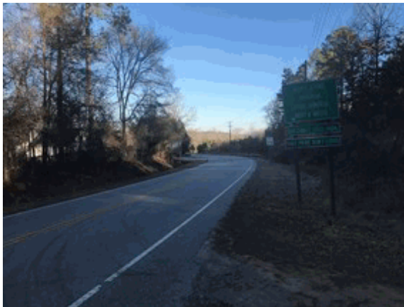
Lost Creek Drive Facing North
