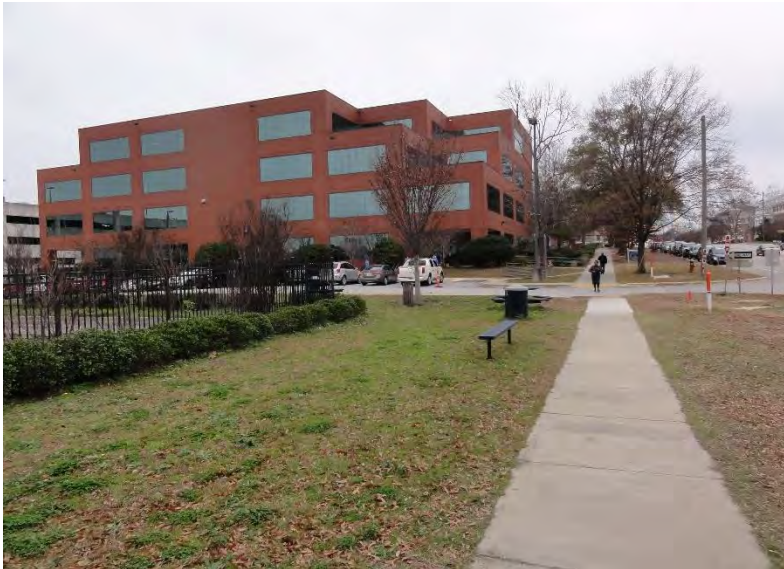
168 of 335 Harden Street sidewalk approaching preferred marker location
