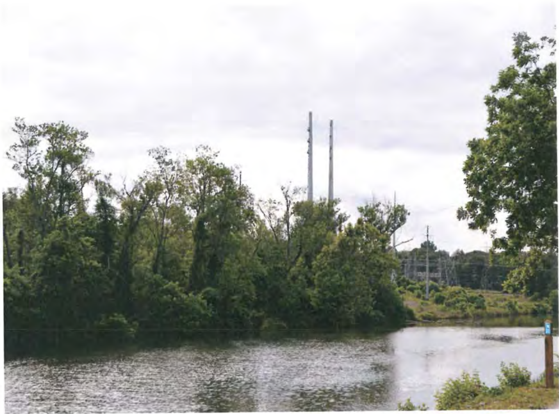
23) Photo facing the proposed tower from the Three Rivers Greenway. Balloon Visible
