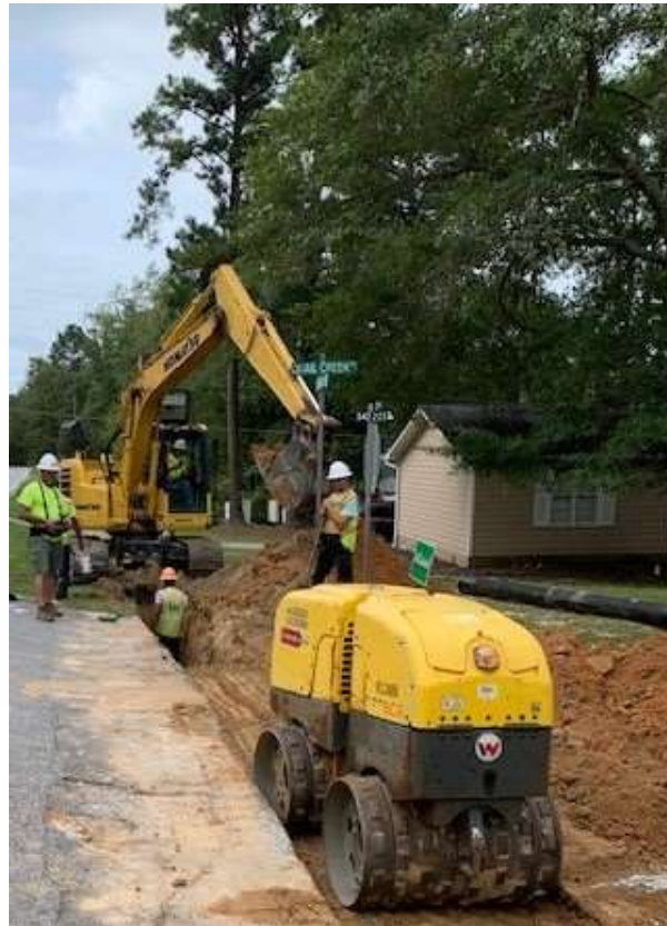
Photo 4: Force main install
