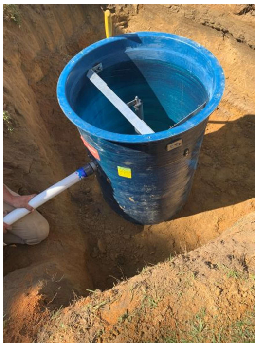
Photo 4: Grinder pump install
