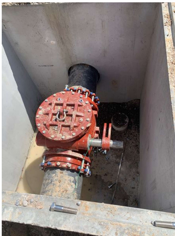
Photo 2: Valve install
