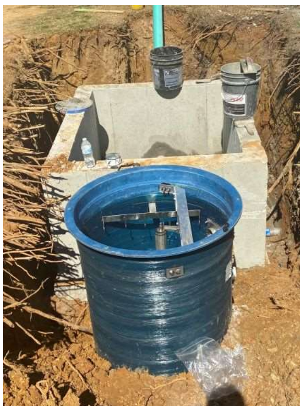
Photo 3: Grinder system install
