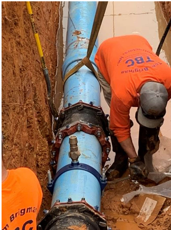
Photo 3: Valve install
