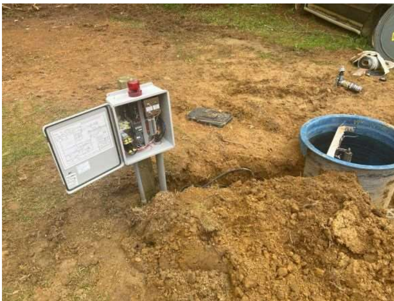
Photo 3: Grinder system install
