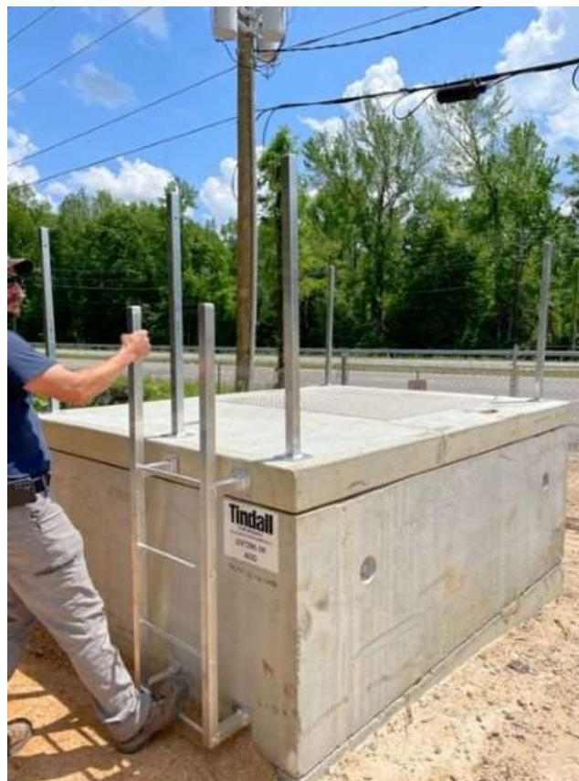
Photo 1: Pit safety access
