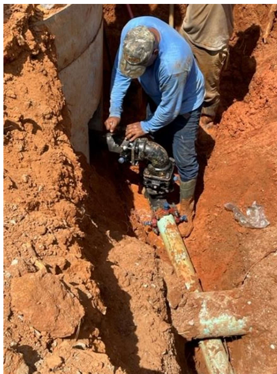
Photo 4: Myers Creek connection
