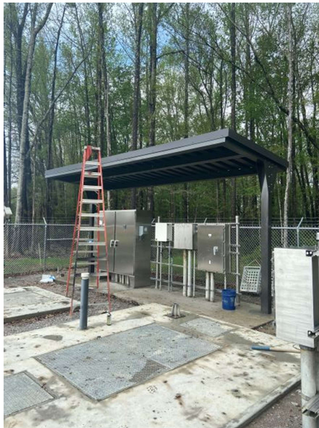
Photo 2: Gadsden pump station
