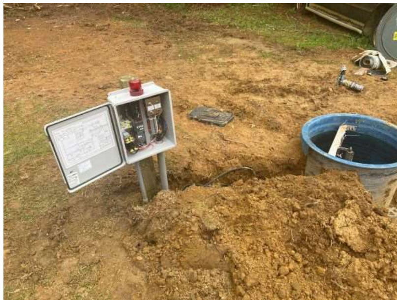
Photo 3: Grinder system install
