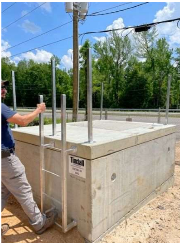
Photo 1: Pit safety access
