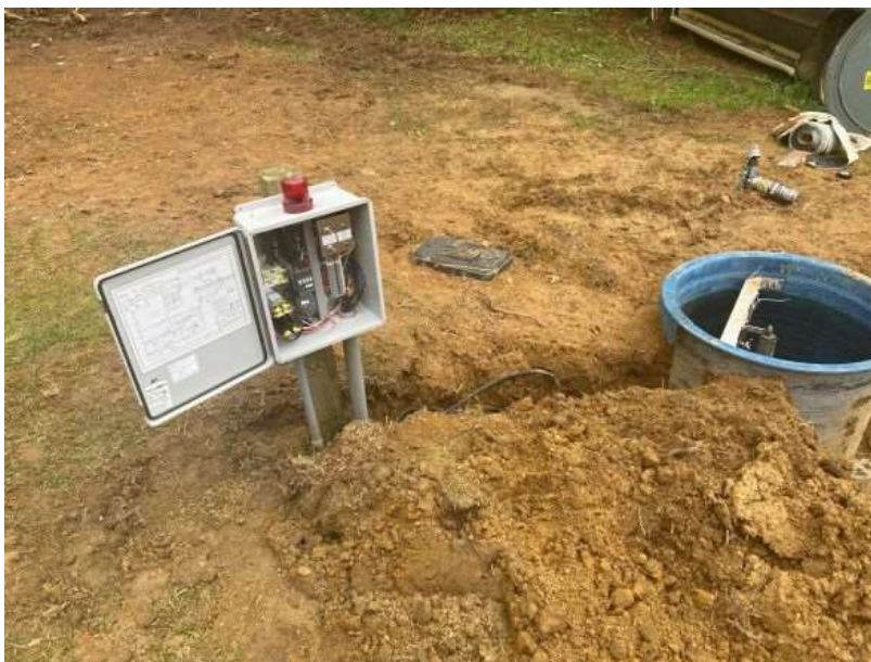
Photo 3: Grinder system install
