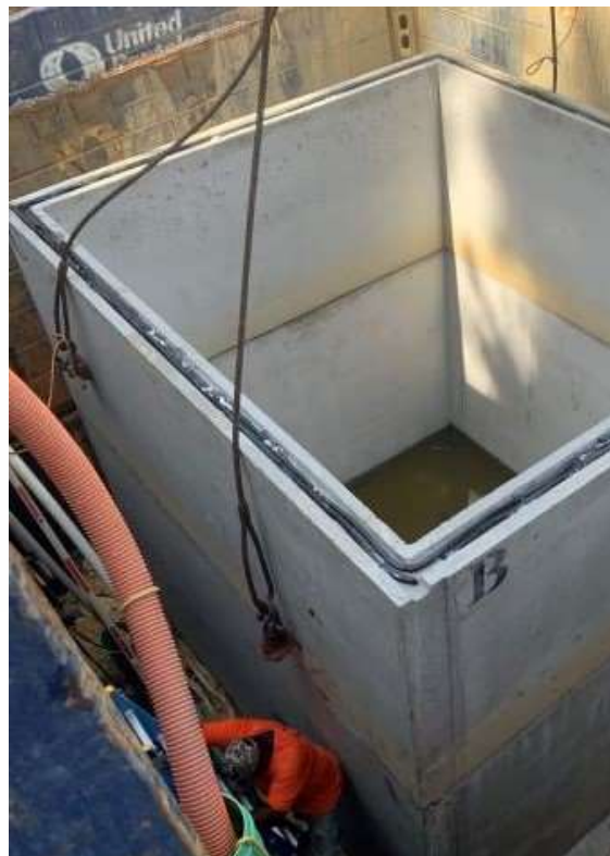
Photo 1: Wet-well install
