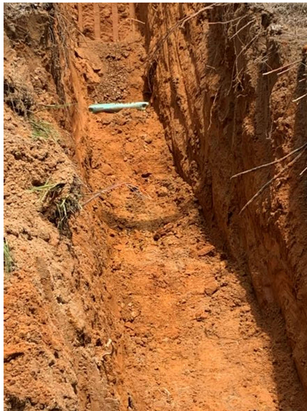
Photo 3: Service connection install
