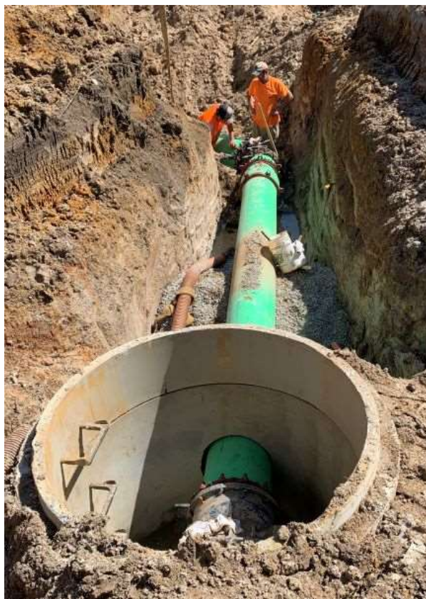
Photo 2: Valve install
