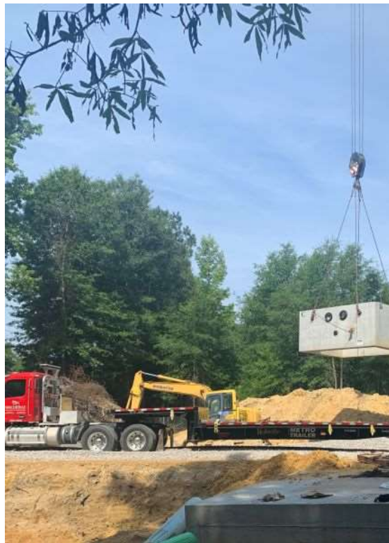
Photo 1: Wet-well install
