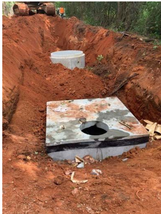
Photo 1: Check Valve Pit
