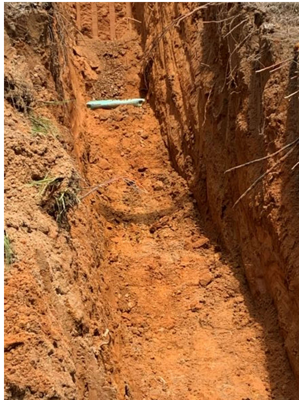
Photo 3: Service connection install
