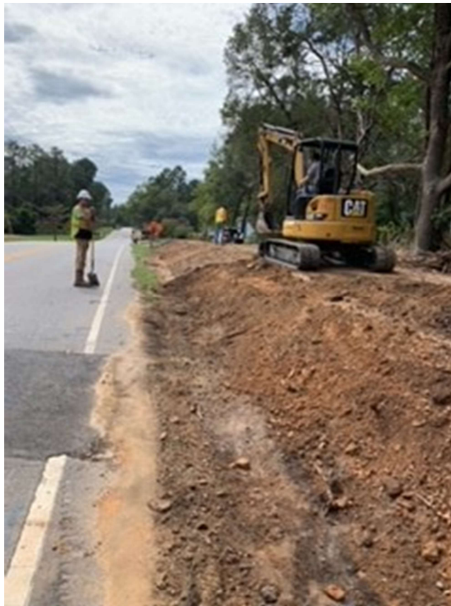
Photo 4: Force main install
