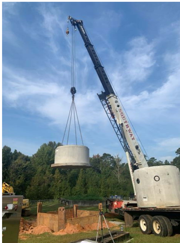
Photo 1: Wet-well install
