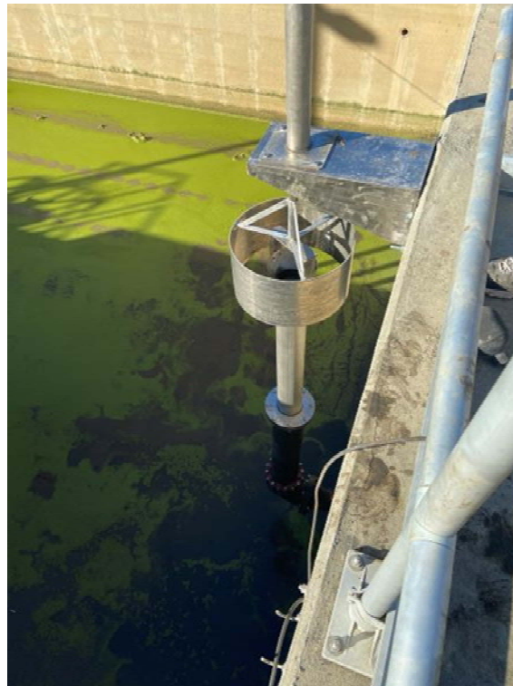
Photo 2: Telescopic valve install
