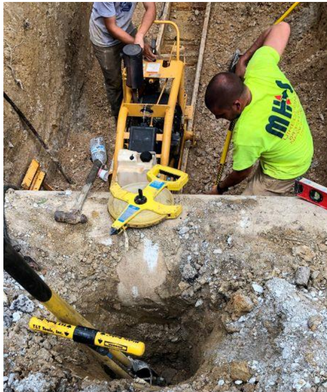
Photo 4: Bore under storm drain
