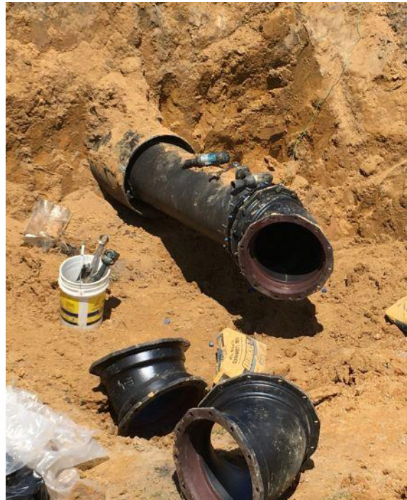
Photo 1: Pipe install in casing
